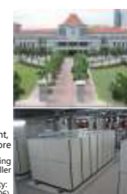
US Embassy in Japan, Tokyo Modular magnetic levitating centrifugal chiller Cooling Capacity: 1600ton (2007)
