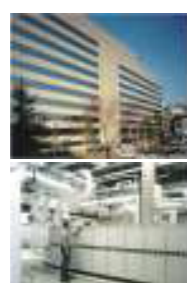
US Embassy in Japan, Tokyo Modular magnetic levitating centrifugal chiller Cooling Capacity: 1600ton (2007)
